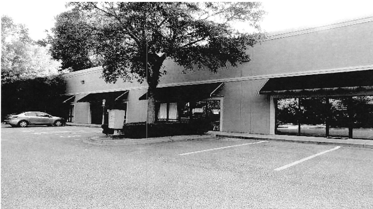
View of existing building
